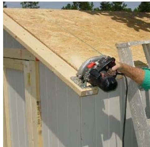
Trimming the Fly Rafter
