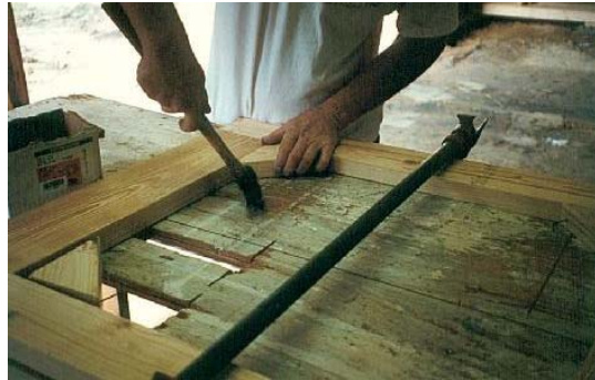
Nail the corner blocks in place.
