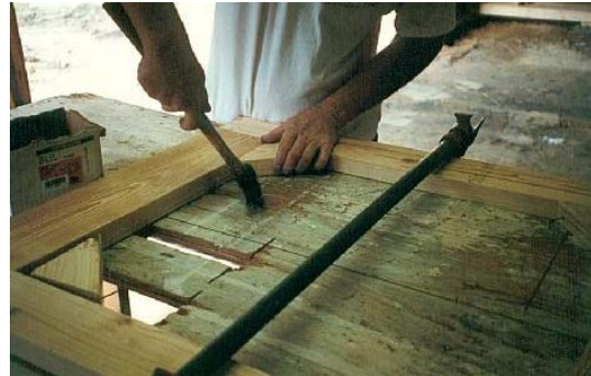
Nail the corner blocks in place.
