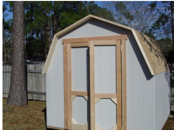
Front Fly Rafters Installed
