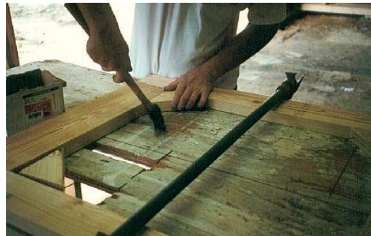
Nail the corner blocks in place.
