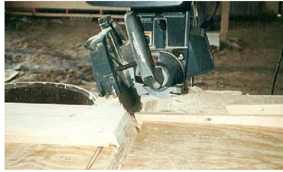
Sawing the fly rafters
