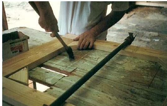
Nail the corner blocks in place.
