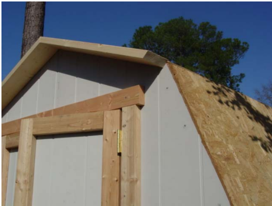
Installing the Fly Rafters
